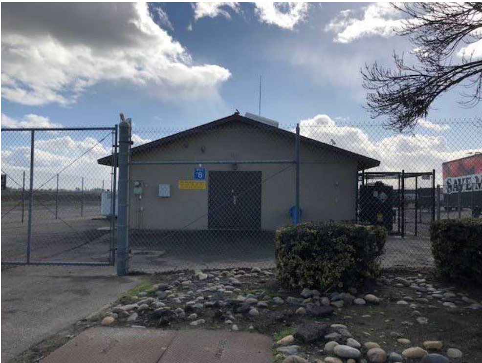
PHOTOGRAPH 3.1-5: GROUNDWATER SUPPLY WELL 8
