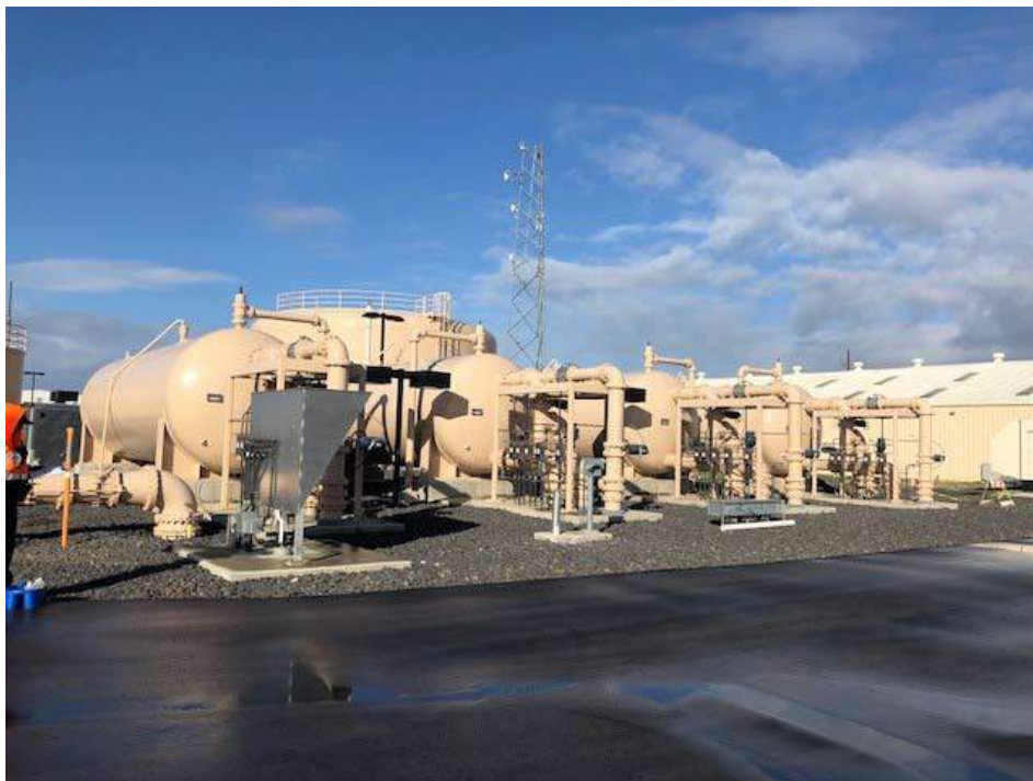
PHOTOGRAPH 3.1-2: LOUISE AVENUE WATER TREATMENT FACILITY
