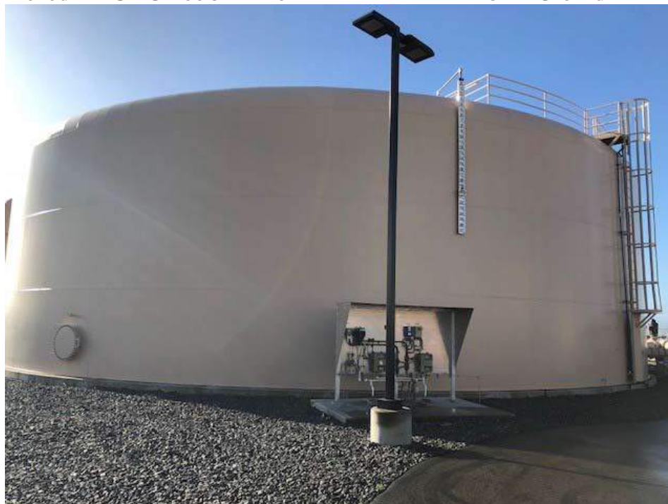
PHOTOGRAPH 3.1-3: LOUISE AVENUE WATER TREATMENT FACILITY STORAGE TANK
